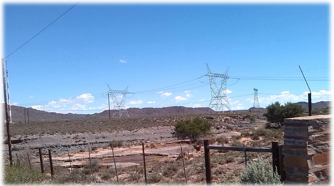
Concerns about close proximity of lines to farm infrastructure
